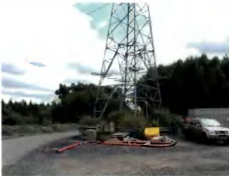
Plate 7: Existing tower located within Intel lands to be decommissioned.
