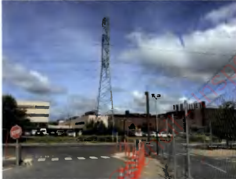
Plate 8: Existing tower in Intel lands towards southern end of OHL to be decommissioned
